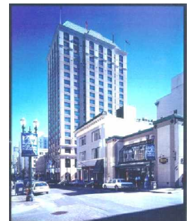
Westin Hotel, Portland, OR, USA. Full height panels with windows preinstalled.
