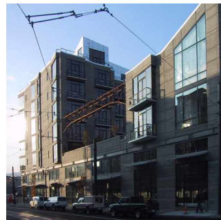
Streetcar, Portland, OR, USA. Full height and spandrel panels.
