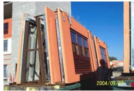
Panels on truck ready for hoisting and installation
