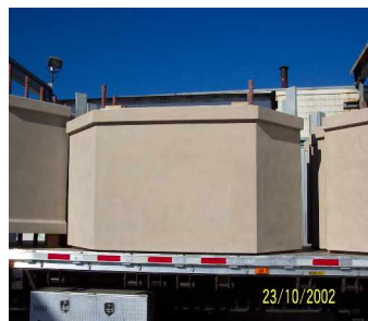
Silver Cloud Inn, Seattle, WA, GFRC spandrel panels loaded and ready to ship to site. These are the bay windows.
