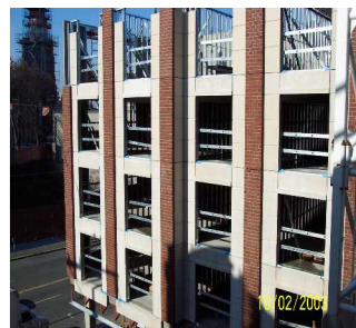
Silver Cloud Inn, Seattle, WA, panel installation
