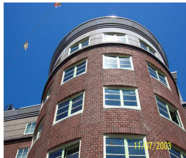
Silver Cloud Inn, Seattle, WA, USA, curved full height and spandrel panels
