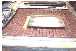
Laid down brick in curved mold
